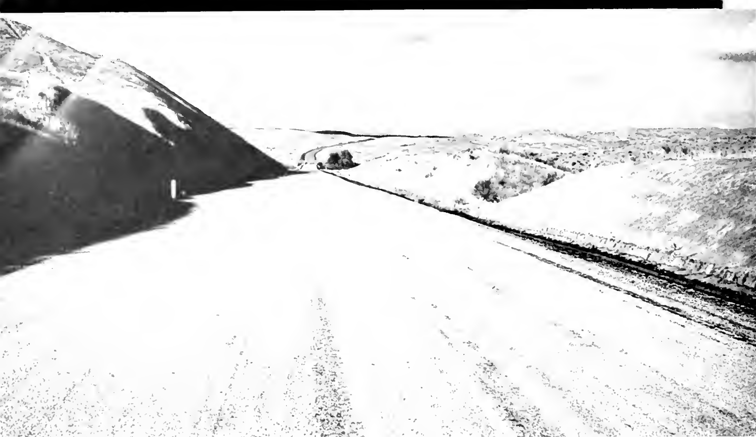
Looking north over completed portion of Ducor Cutoff. Bridge in background is over Poso Creek
